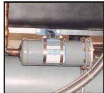
Typical filter-drier Figure 6.2D
